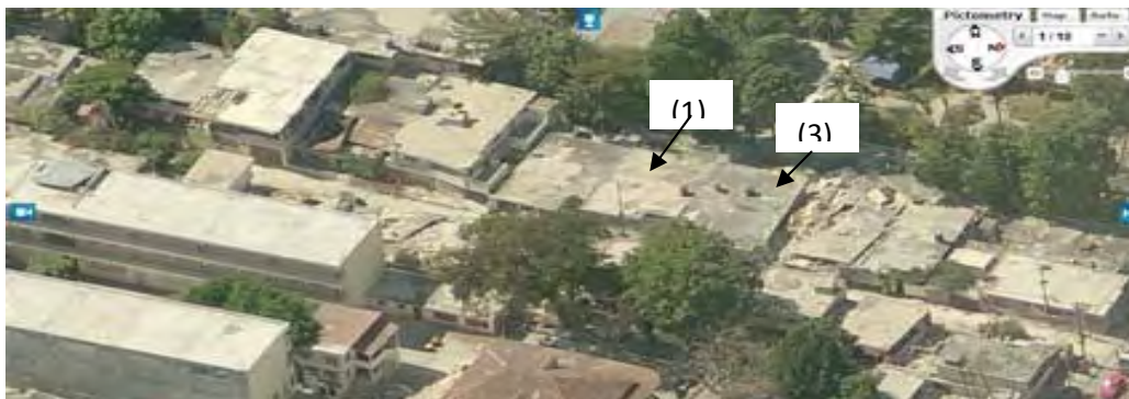
Figure 11 Buildings (1) and (3) in Figure 10 as seen in Pictometry.
